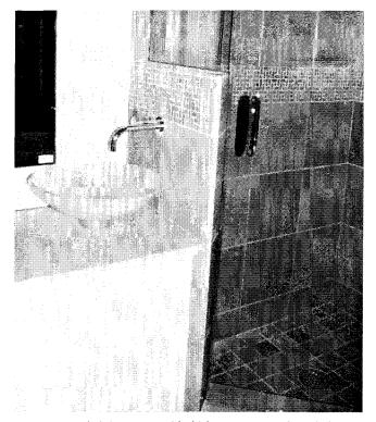
Fig. 5. Stone tiled shower set with thick set mortar and sanded grout.
