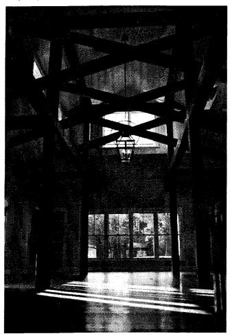
Fig. 4. Living room truss made from recycled timbers.
